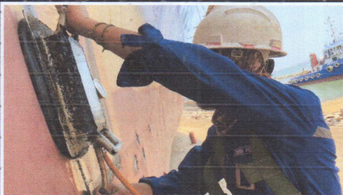
Leak test area replating
