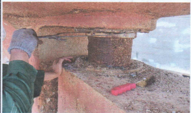
Clearance Check Rudder Stock
