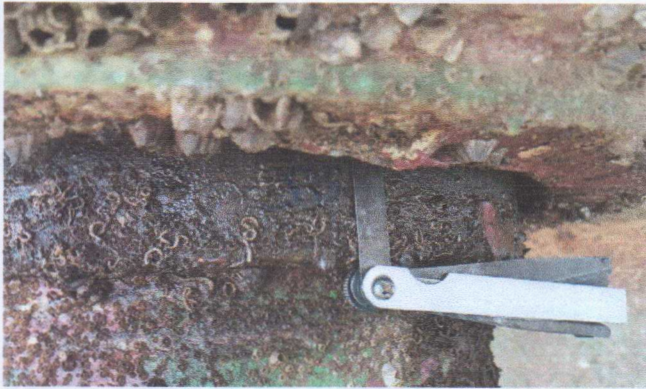
Clearance Check Rudder Stock
