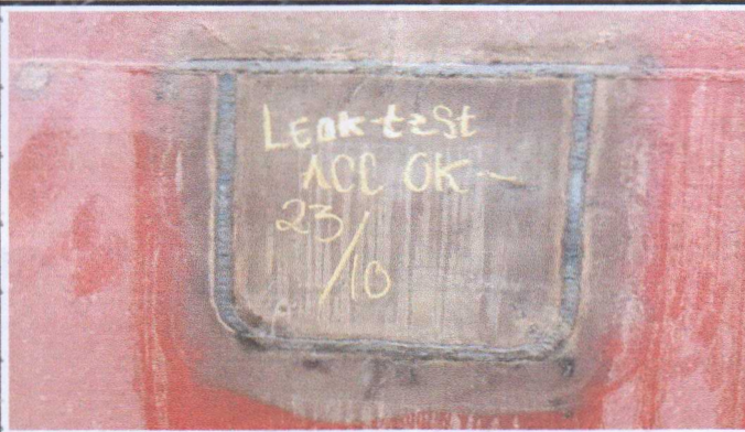
Leak test area replating
