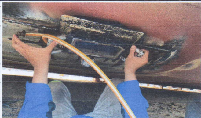
Leak test area replating
