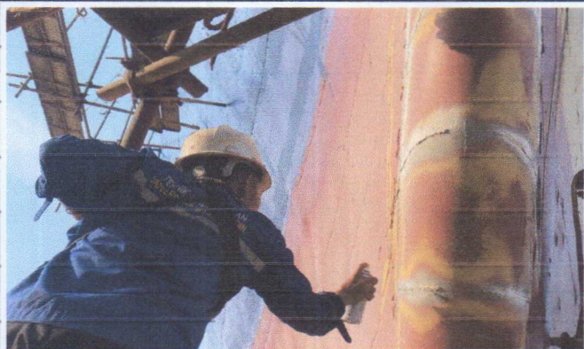
Leak test area replating
