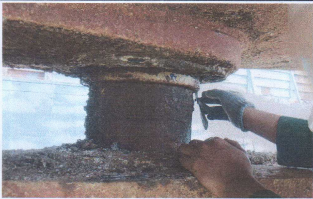
Clearance Check Rudder Stock
